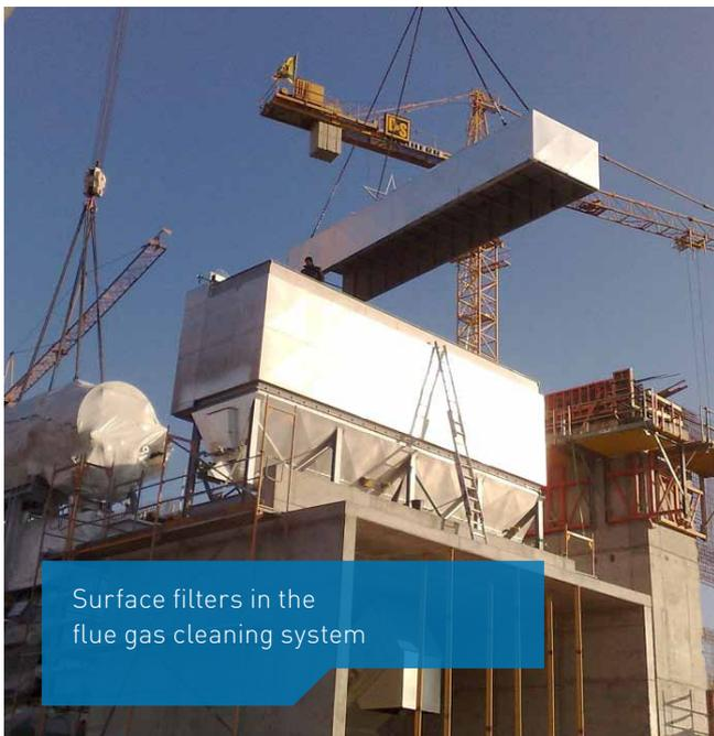
Surface filters in the flue gas cleaning system
